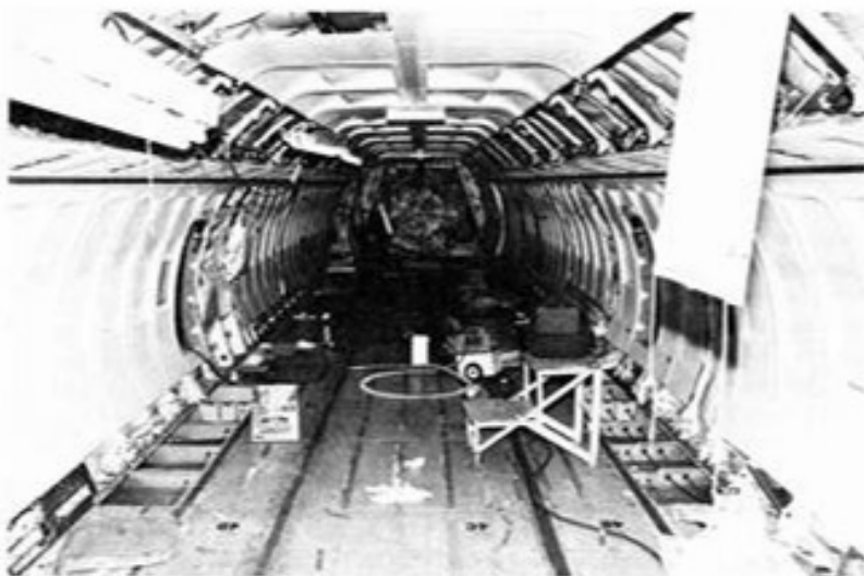
The interiors are completely stripped out.
